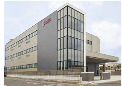
A new factory of IFS started operation in April, 2021.
